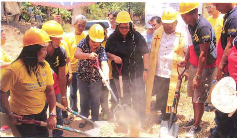
NEA Administrator Edita S. Bueno (third from L), Coron Mayor Clara "Fems" Reyes (fourth from L), and BISELCO General Manager Ruth Galang (leftmost) lead the laying of time capsule for the inauguration of the Barangay Lajala submarine cable project. The 1.9 km submarine cable will deliver power from Barangay Poblacion 5 to Uson Island, Barangay Lajala, and is expected to be operational by the first week of August 2016.
